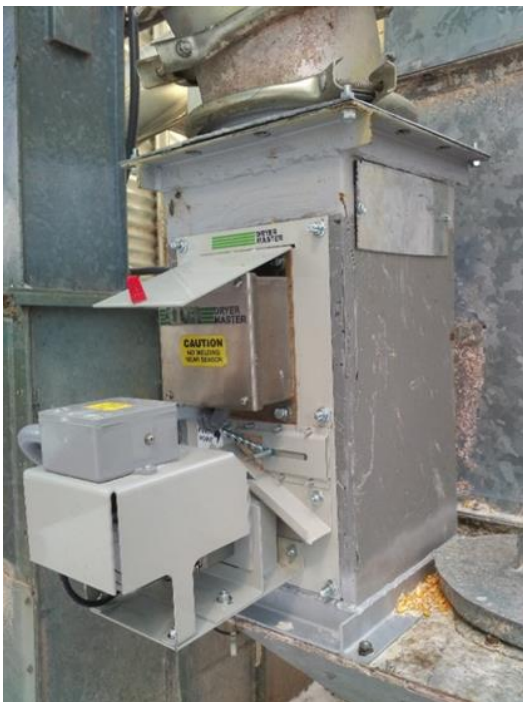
Figure 19 - In-line Chute installation example
